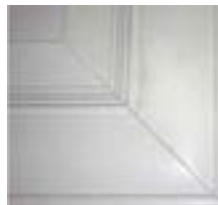
REPRESENTATIVE OF ACCEPTABLE MITER JOINT
